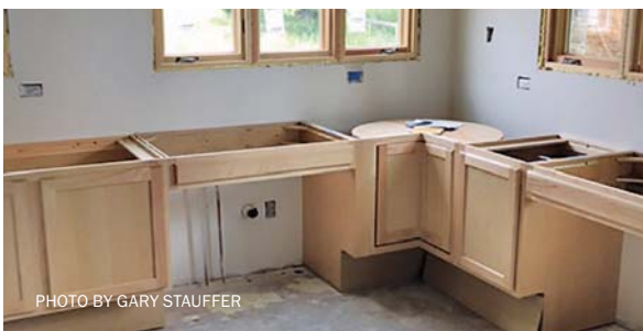
New cabinets being installed in the farmhouse
