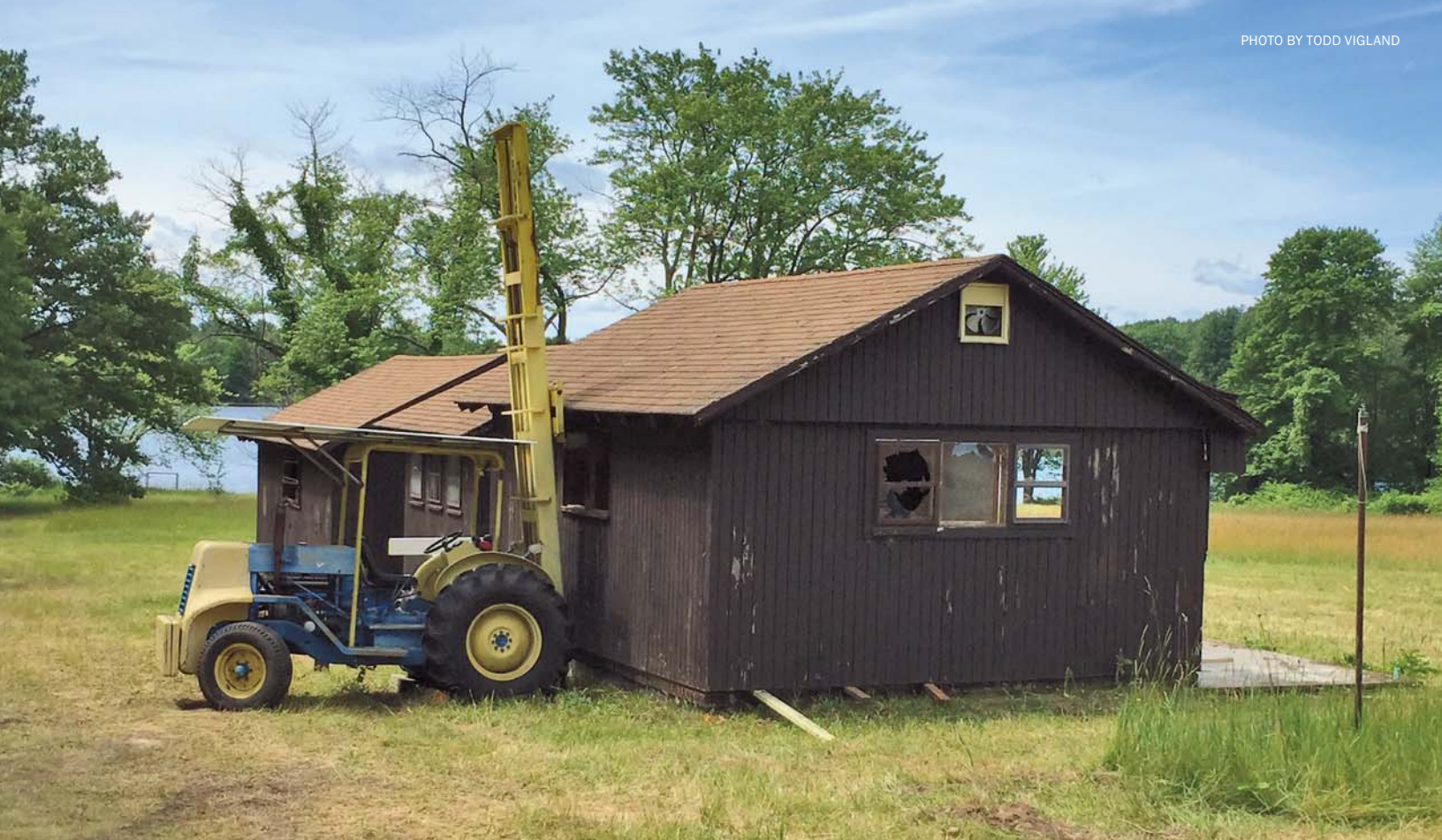
Cabins being removed from the former Camp Maplehurst
